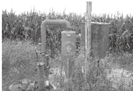
(B) The well was drilled in 2010 with the financial help from the country (Depth 70 m)
