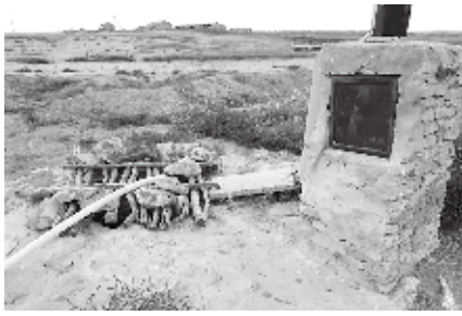
(A) The well was drilled in 1959 (Depth 23 m)
