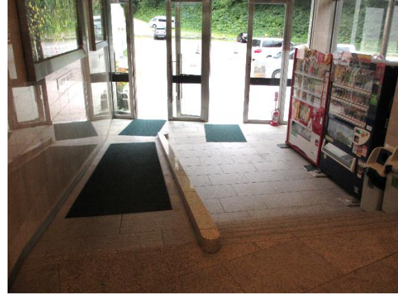
Figure 5.2.56: The accessible entrance at the back of the Kurodake Ropeway Station
