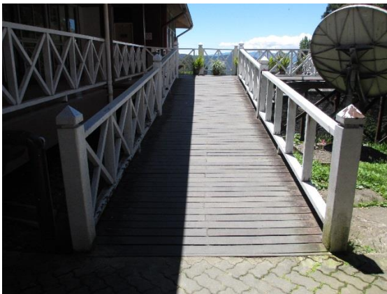
Figure 5.2.17: The slope going up to the visitor center.
