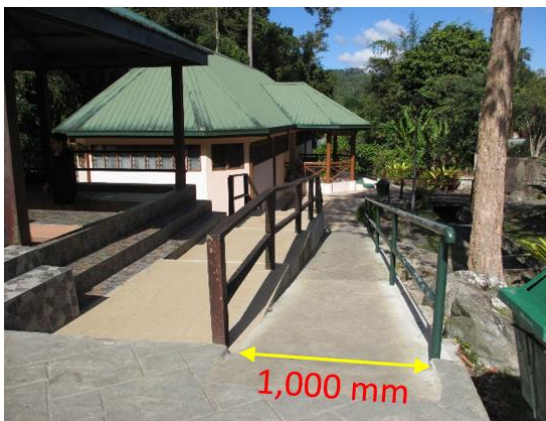
Figure 5.2.49: The ramp to the changing room and public toilet
