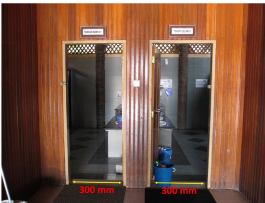
Figure 5.2.5: The toilet at the center
