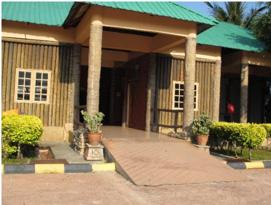
Figure 5.2.3: The slope to the visitor center
