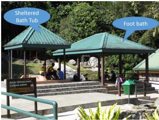
Figure 5.2.47: The staircase to the sheltered bath tub and foot bath.
