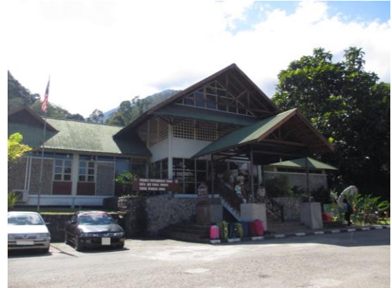
Figure 5.2.34: The administration office
