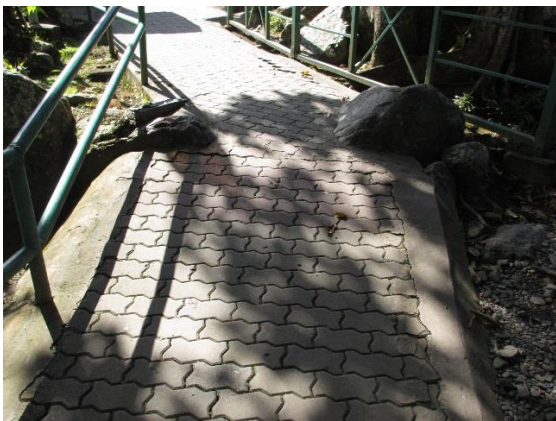
Figure 5.2.41: The uneven, small width path.
