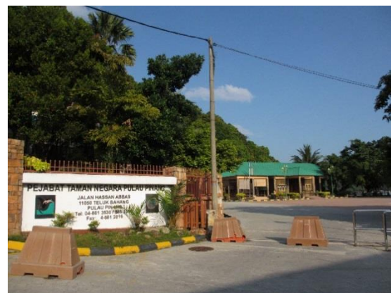
Figure 5.2.2: The main entrance of the PNP
