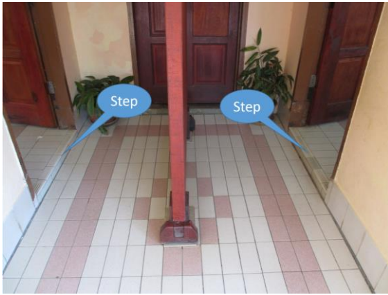
Figure 5.2.51: The narrow entrance space and step.
