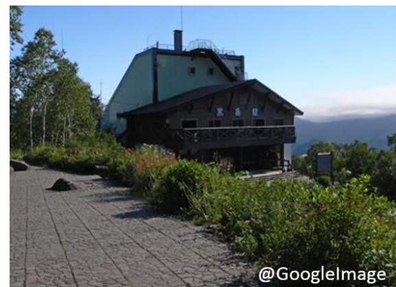
Figure 5.2.60: The rather uneven paved path (with gaps)
