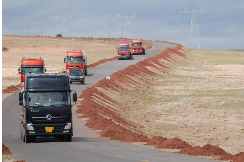
The National Highway 109, Wudaoliang area.
