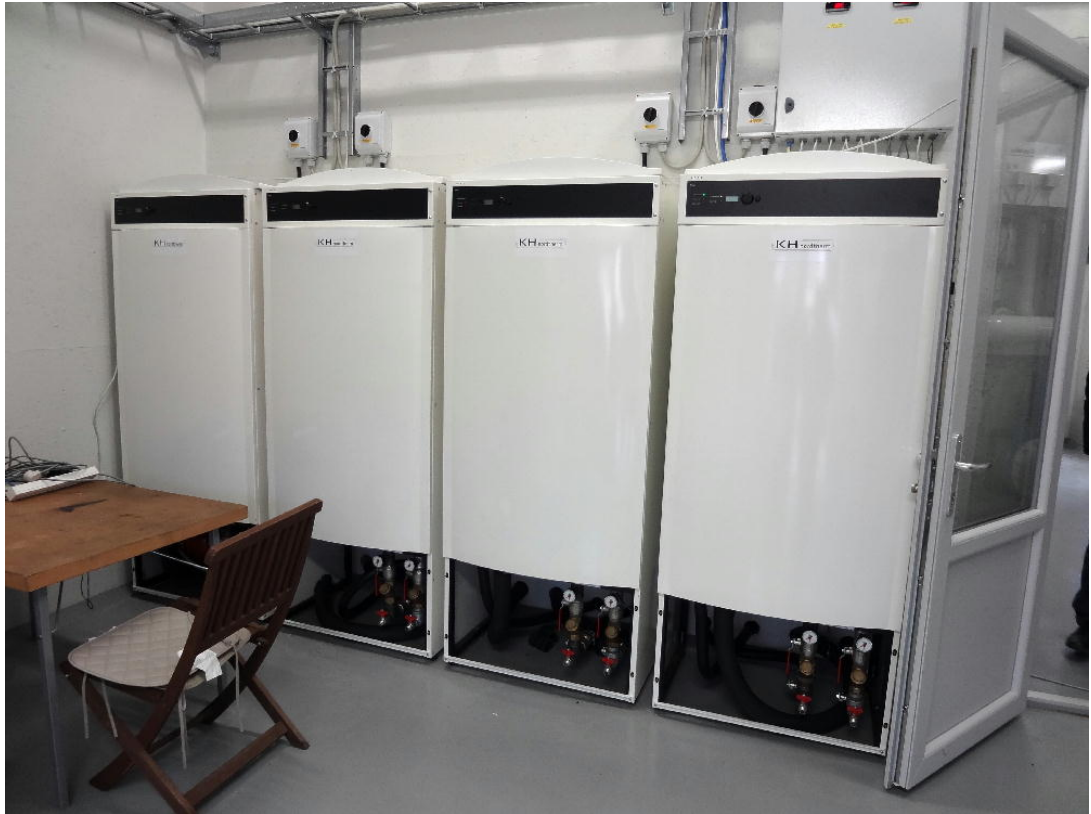
Photo 5-2. Heat pump for recovering heat from the digested slurry (ComBigaS, Photo by Nakayama)
