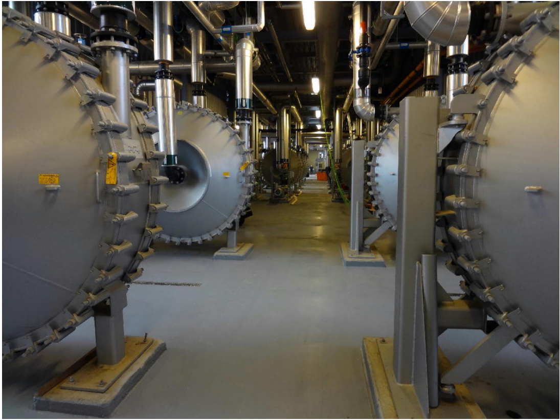
Photo 5-3. Heat exchanger for recovering heat from the digested slurry (Maabjerg bioenergy, Photo by Nakayama)
