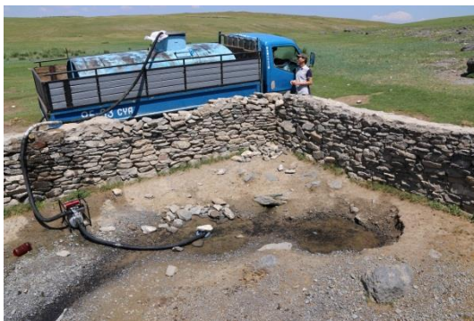
Water pumping from spring
